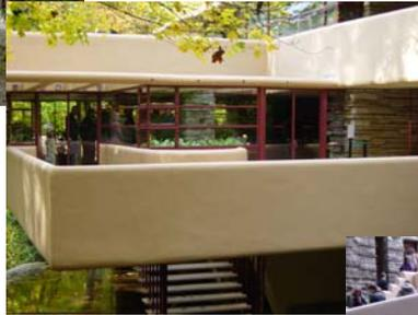
beam, supported only at one end. Wright actually anchored most of the cantilevers of Fallingwater into boulders
